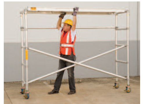
3. Install platform at desired height.
